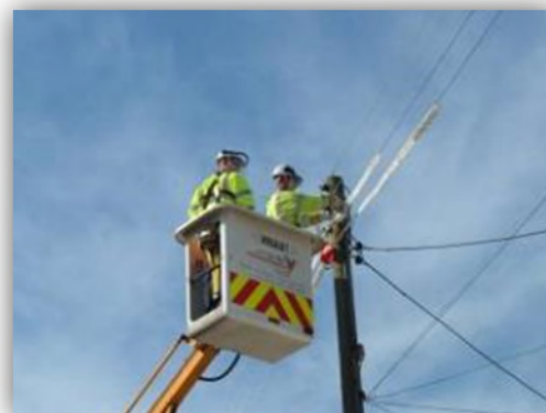
Fitting low energy LED lamps
